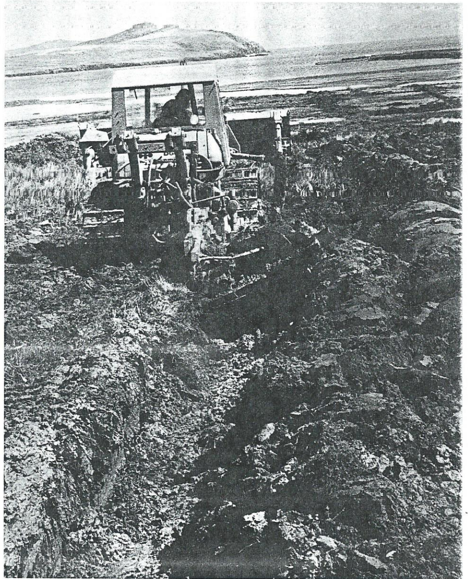
Deep ploughing with a swamp bulldozer and five ton plough. The Co-Op have reclaimed more than 6,000 acres of land in the last eight years.
